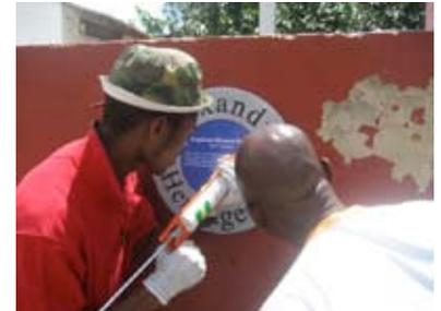
Insert installed and sealed
